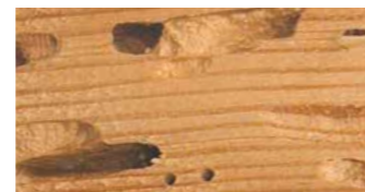
· DAMAGE Exit hole: oval > 1/4 inch Bore dust: colored cylinder Timber attacked: sapwood of softwoods
